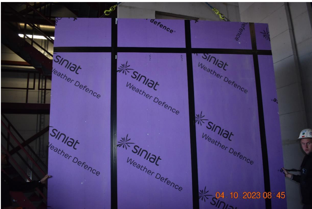
Photo No. 2 Prefabricated wall front side.
