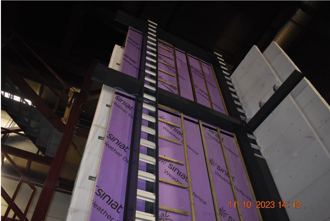
Photo No. 15 Vertical steel cassettes are mounting.
