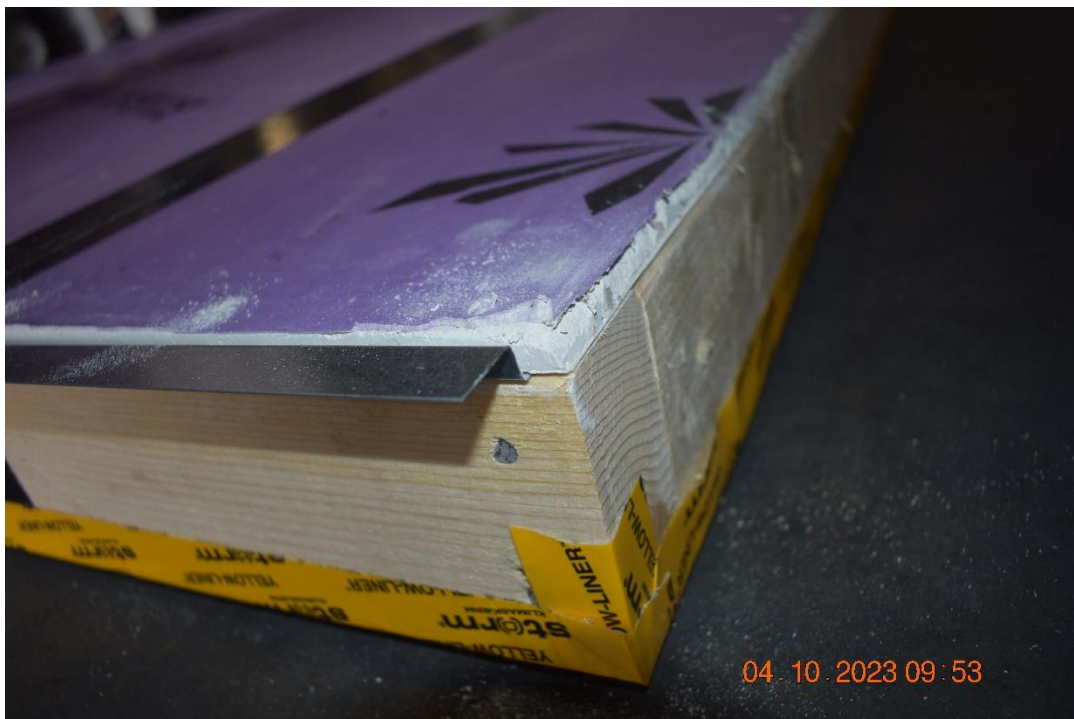
Photo No. 4 z-profile between the construction wood and weather defence.
