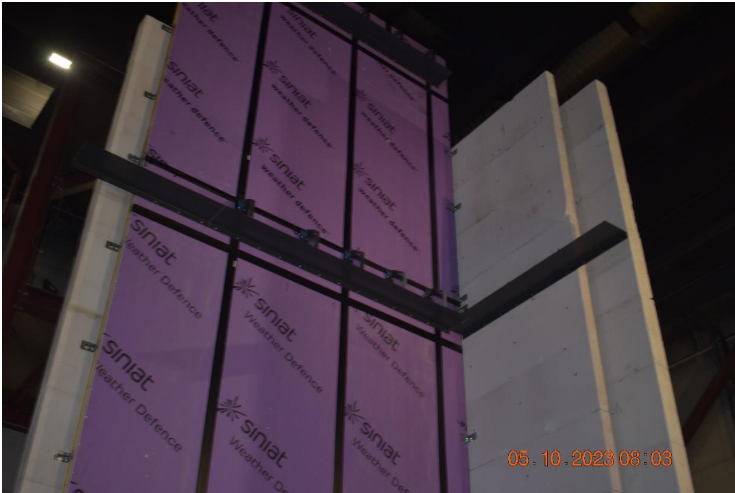
Photo No. 7 Bracket profiles mounted on the wall and flame deflector.
