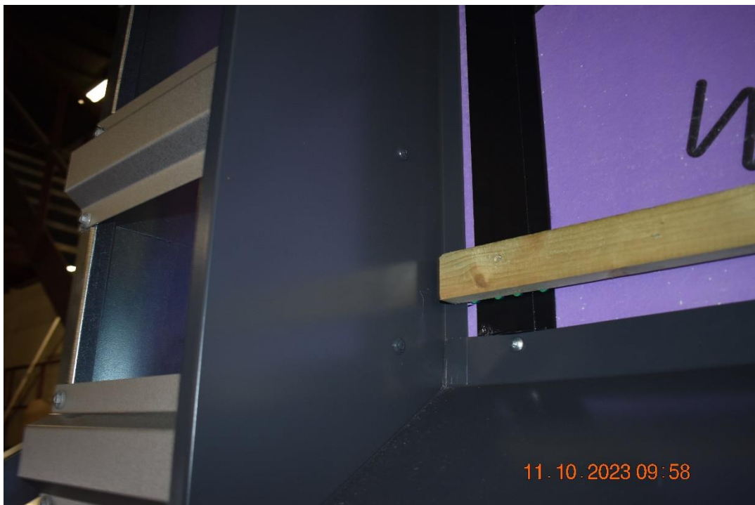
Photo No. 14 Vertical side coverings were mounted on the C-profile.
