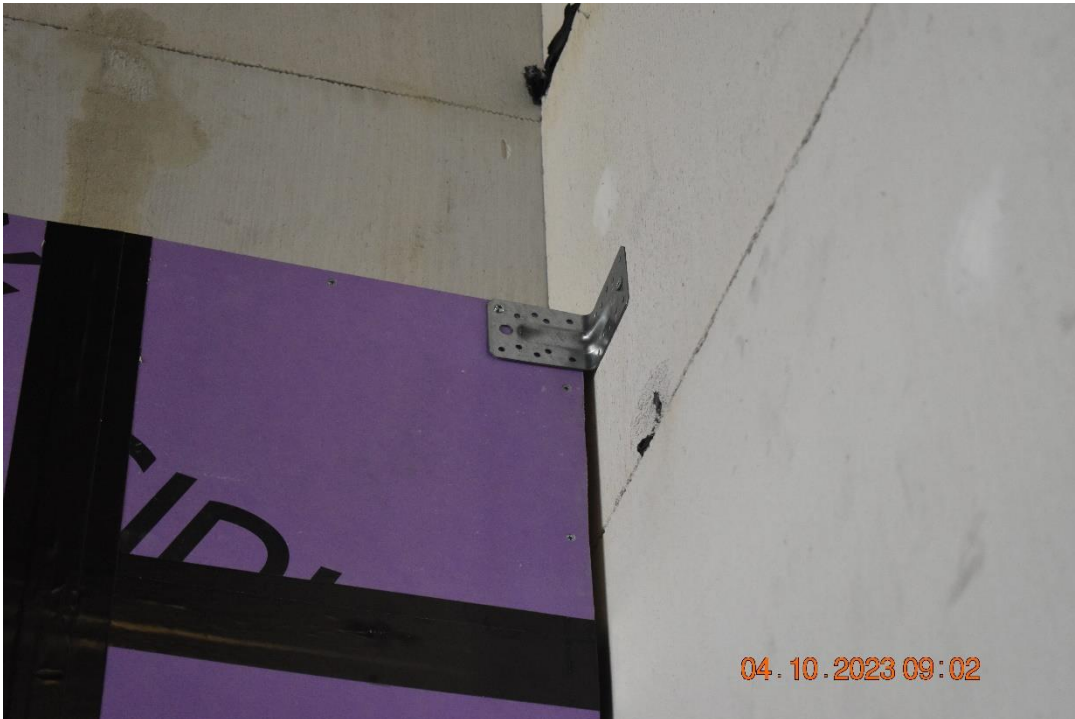
Photo No. 5 Steel angle to mount the wall on façade rig.
