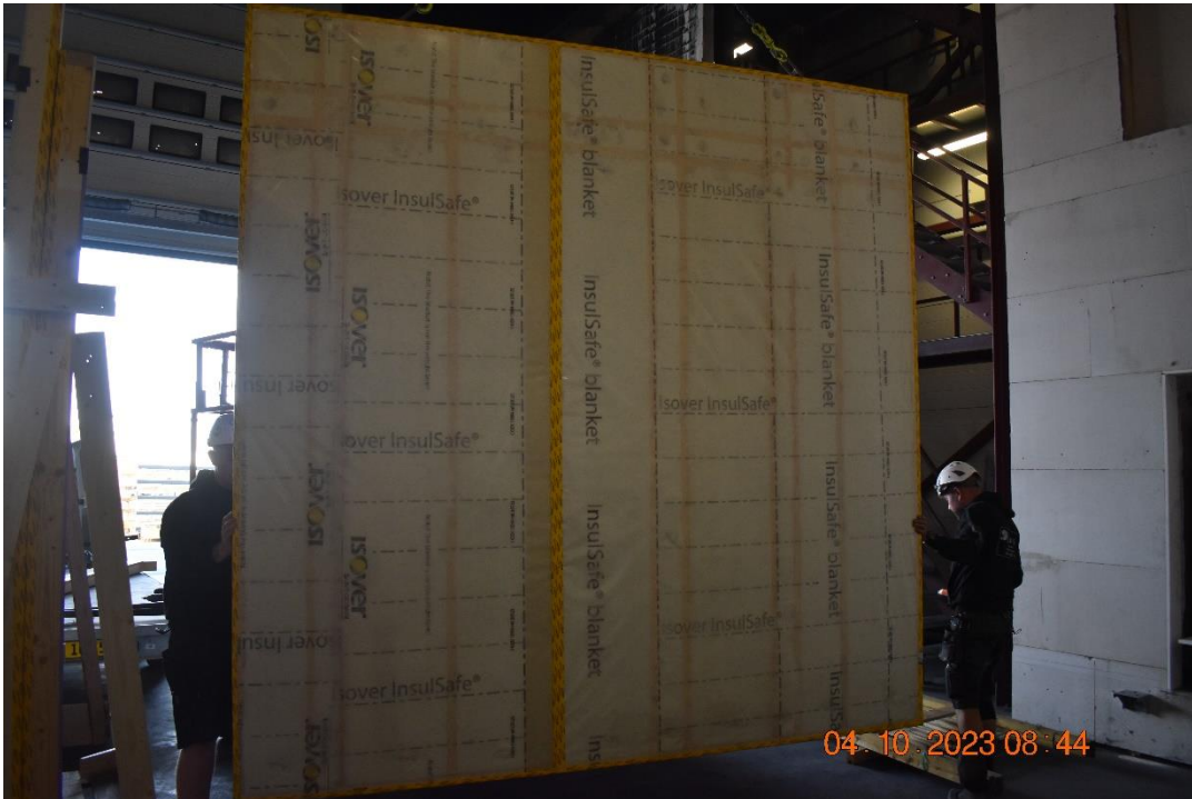
Photo No. 1 Prefabricated wall back side.
