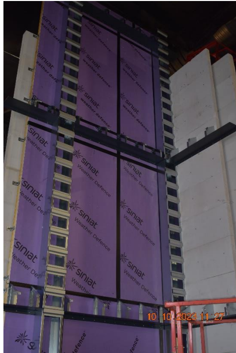
Photo No. 11 Hat profiles were mounted on the C-profiles.
