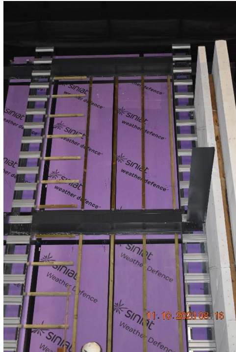
Photo No. 13 Horizontal flame deflectors are mounting.
