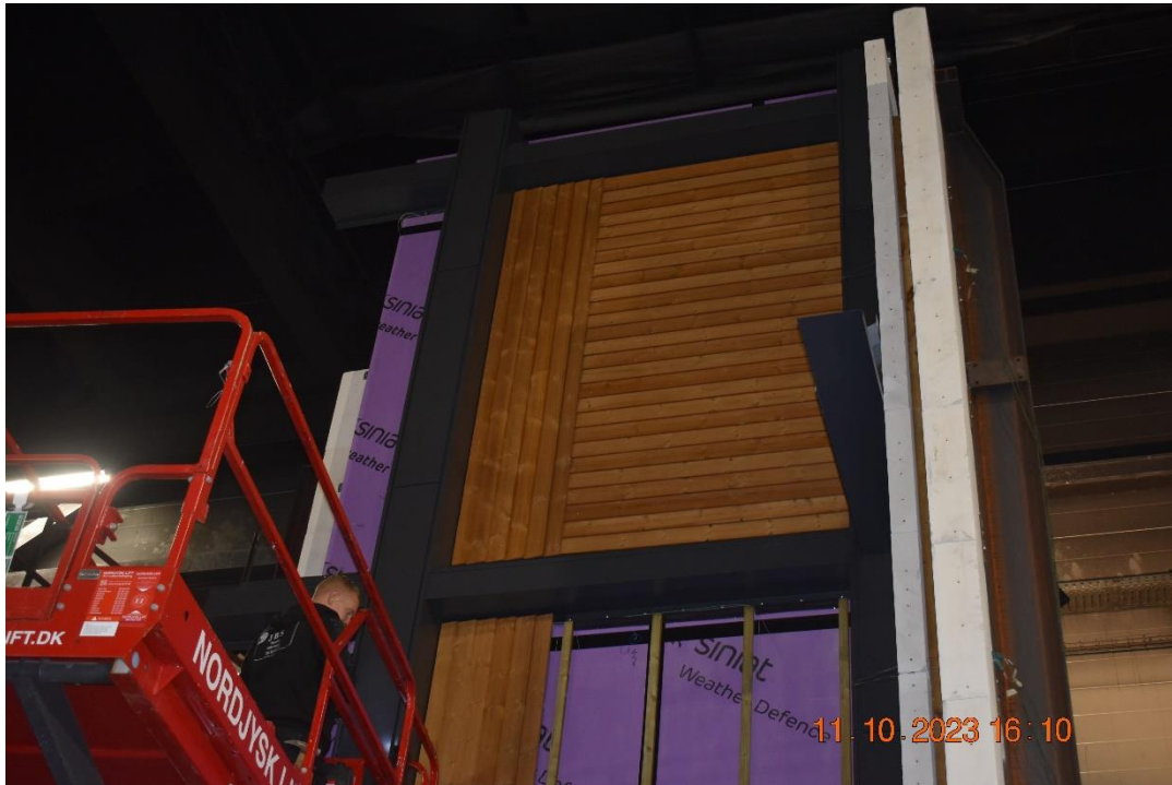
Photo No. 17 Cladding is being mounted.
