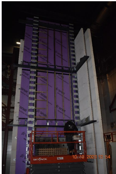
Photo No. 12 Formworks were mount on the wall.
